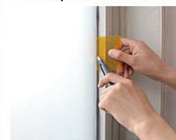
Cut off excess around the edges
